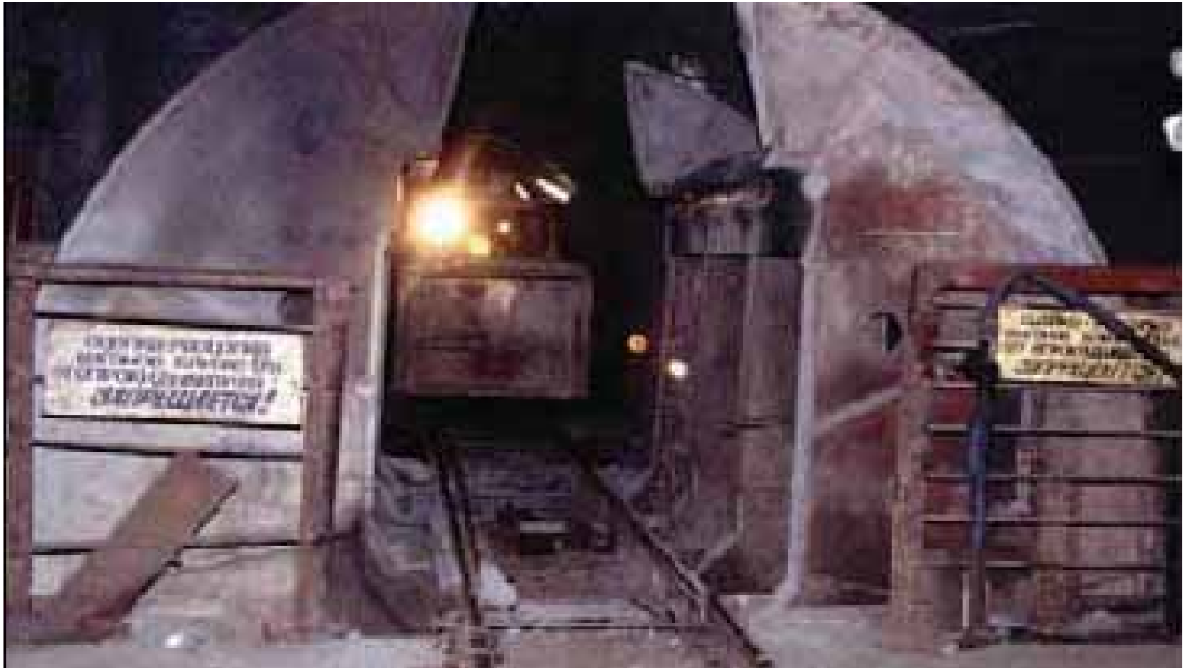
Ore Transfer Section Norilsk Orkyabyrsky Mine
